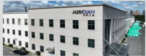
Meridian LT: Located in Pinghu, Zhejiang province for the production of all injection molded plastic products.
